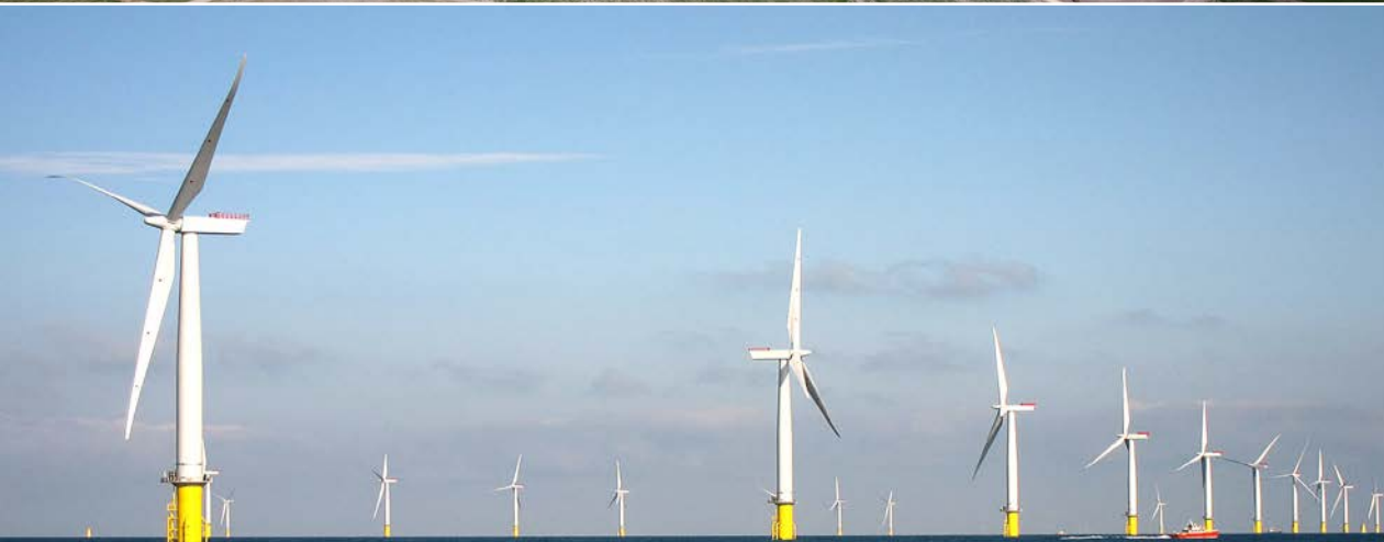
London Array, the world's largest offshore wind farm (630 MW)
