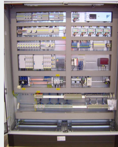
Cool Expert control cabinet
