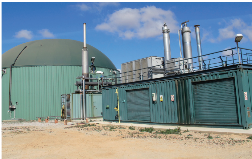
Figure 3.1.5.2: A biogas-producing anaerobic digestion plant. | Source: RENAC.
