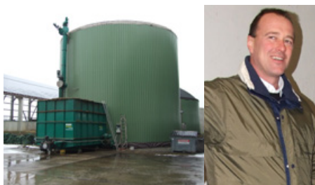
Hubert Miller has been an organic arable farmer in Schmiechen, Germany, since the 1980s. For the last six years he has run a 350 kW biogas plant with an extra high fermenter and vertical stirring. He uses a substrate mix containing up to 98% cover grass from about 40 organic farms. Photo: F. Gerlach, MEP
